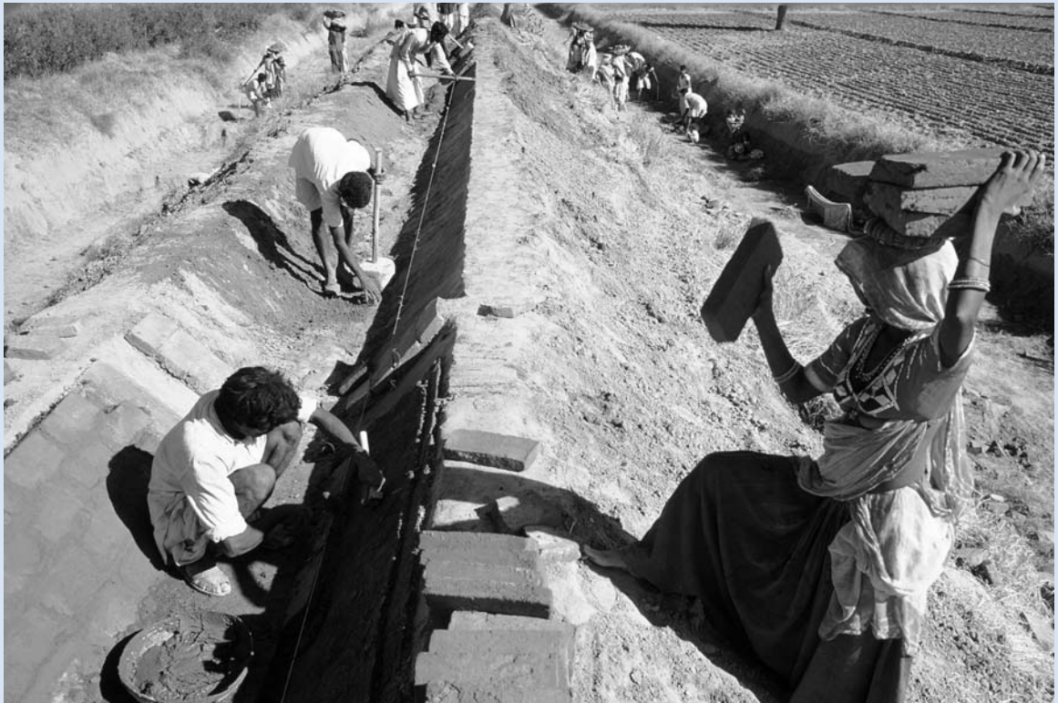
Building a canal for irrigation in India. Photo by Ray Witlin, courtesy of World Bank Photo Library.
