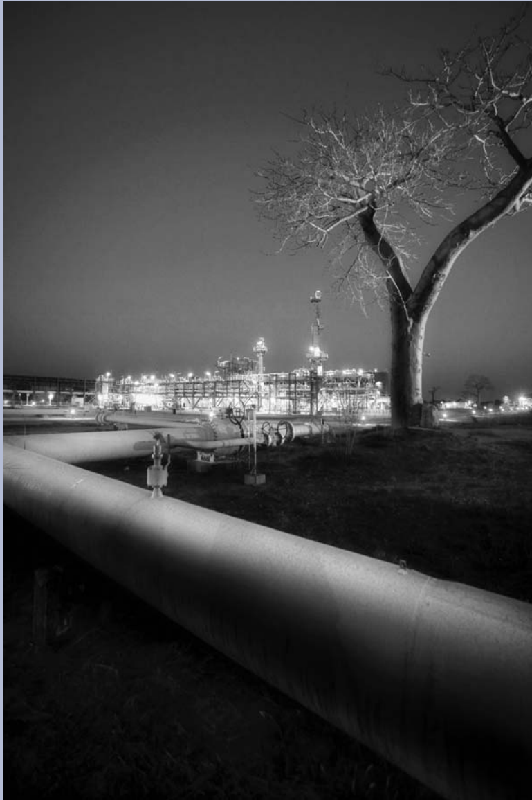
Complex cross-border projects represent high-risk endeavors that can benefit from WBG guarantees. Photo courtesy of Sasol, a gas pipeline project guaranteed by MIGA and the World Bank.
