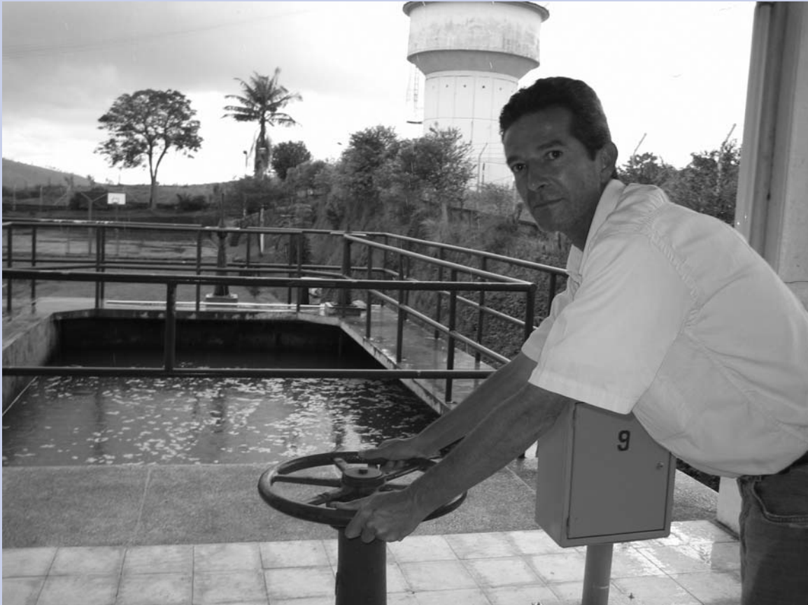
MDP-funded municipal water treatment plant in Pereira, Colombia. Photo courtesy of Roy Gilbert.
