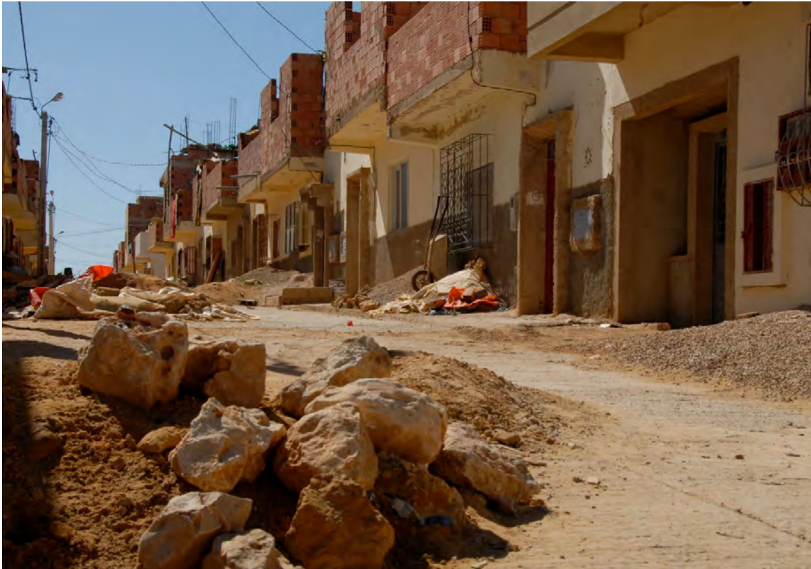
3. New housing being built for ex-bidonvillois in Meknes
